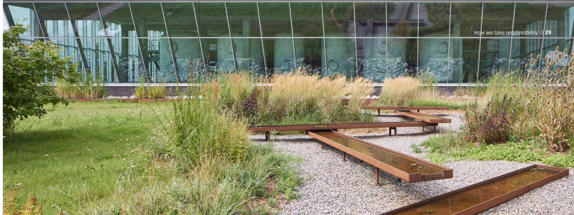
> Køge Waterworks Photo: Gottlieb Paludan Architects
